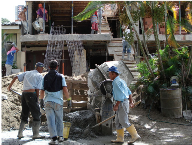
Figure 2. Construction of a Three-Story Apartment Building in Medellín, Colombia
